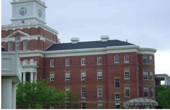
Figure 2.5 Forwood Building, US Soldiers and Airmen's Home
